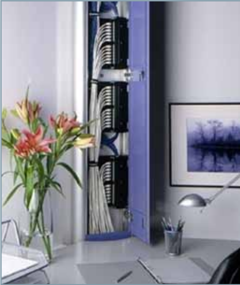
Figure 3. Architectural columns are useful in retrofit applications for hiding cable runs.
