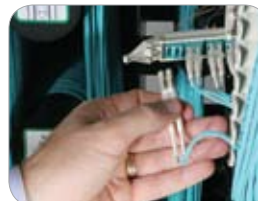
Data Center ODF, MPO Block and Sliding Adapter Pack
